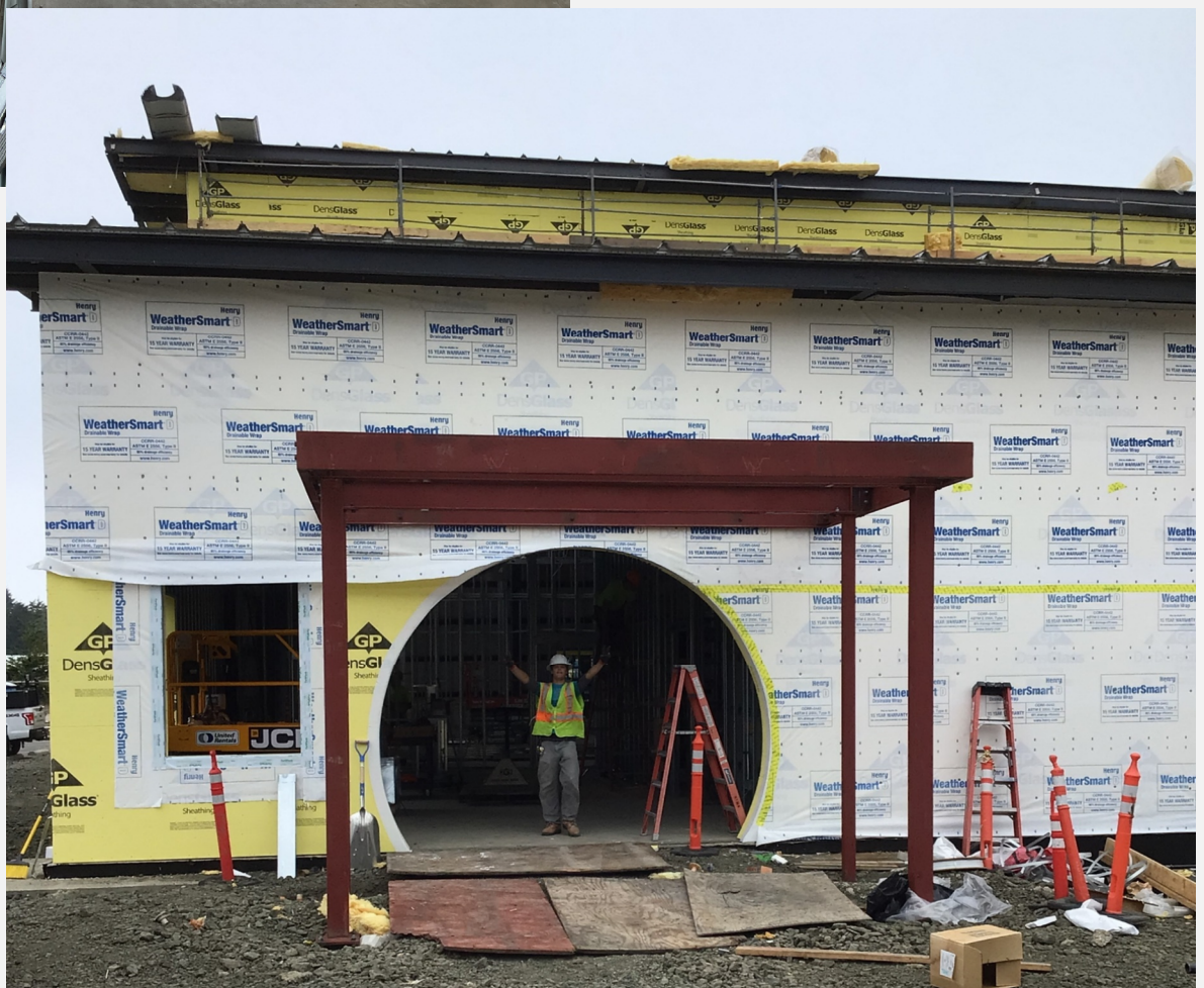
Below: The main entrance framing ready for the new front doors.
