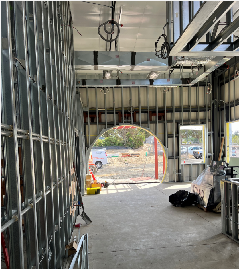
Below: The main entrance framing ready for the new front doors.
