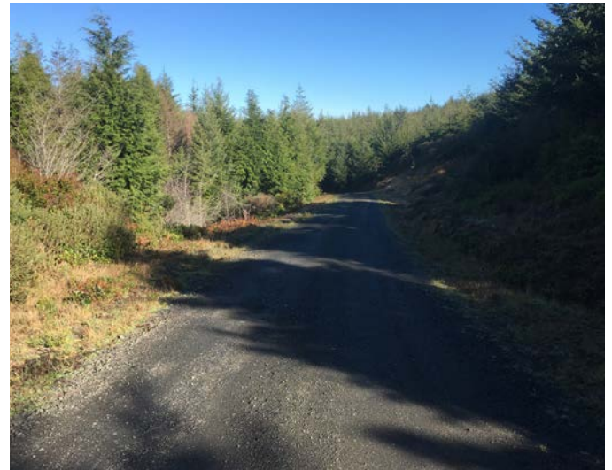
Second Creek Access Road looking north
