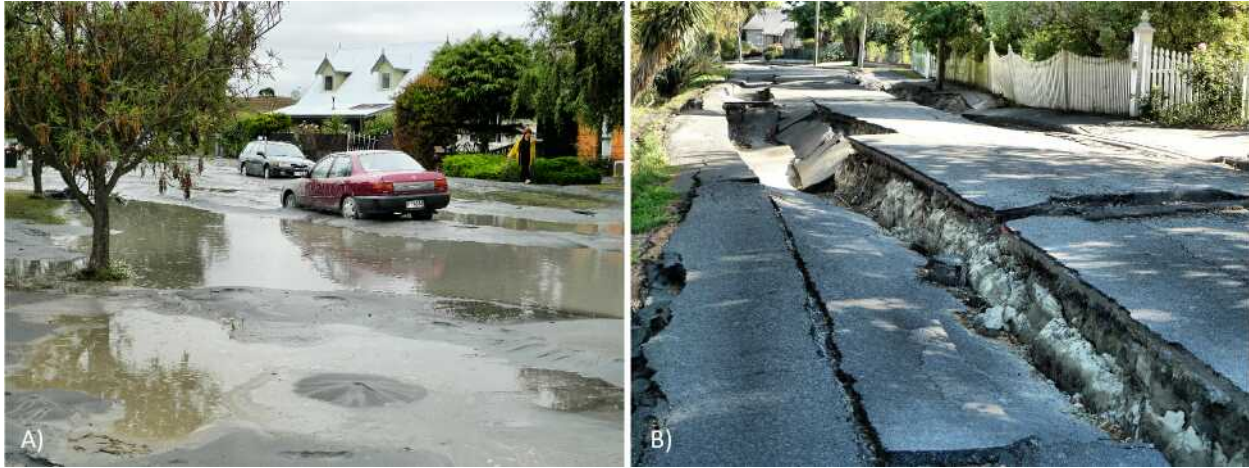
Figure 2-1. Water-saturated sand can turn to quicksand during strong shaking, forming sand boils, ponding, and sunken roads. In these examples, (left) extensive liquefaction occurred along River Road in Christchurch, New Zealand following the February 2011 earthquake, while (right) effects from lateral spreading along numerous Christchurch roads constructed next to waterways resulted in major failures to road infrastructure as roads slumped toward river channels. During a Cascadia subduction zone event, such processes could compromise tsunami evacuation routes as well as the time and speed to safety in areas prone to liquefaction. (Photo credits: Martin Luff, licensed under CC BY-SA 2.0)
