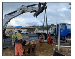
The main shutoff valves for fresh water were installed last week and were flushed today.
