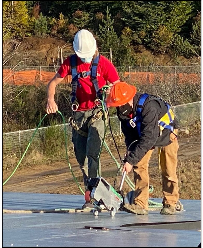
Top: Workers from Rich Rayburn Roofing seal seams in the roof membrane.
