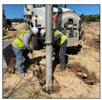
**Above:** Workers use a vacuum truck and a water jet to drill a vertical hole. They're pinpointing the location of a pre-existing utility line, so that excavation won't disturb it. The man on the left uses water to loosen the dirt. The man on the right directs a vacuum nozzle that sucks up the resulting mud. The rig can drill as deep as 16 feet.
