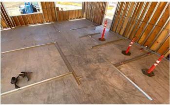
Above, roof joists support plywood sheathing above the medical clinic. Bottom, steel sill plates show locations of interior walls.
