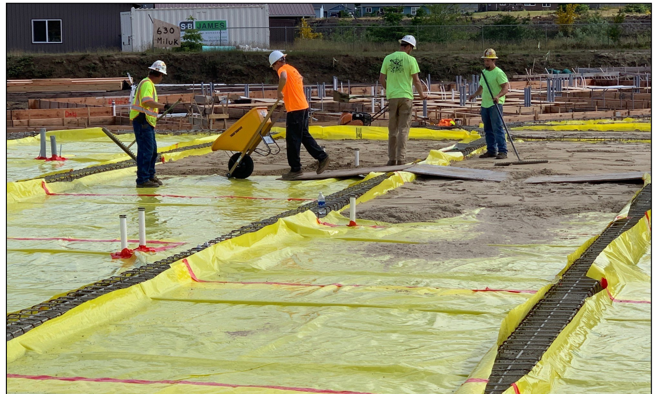
Below: Workers lay down a plastic vapor barrier and a layer of sand in preparation for pouring the concrete slab. The white pipes are stubs of sewer lines. Photos by Lon Matheny
