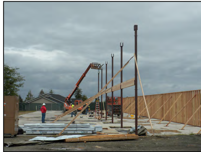
June: Steel posts ensure a sturdy ridge line.
