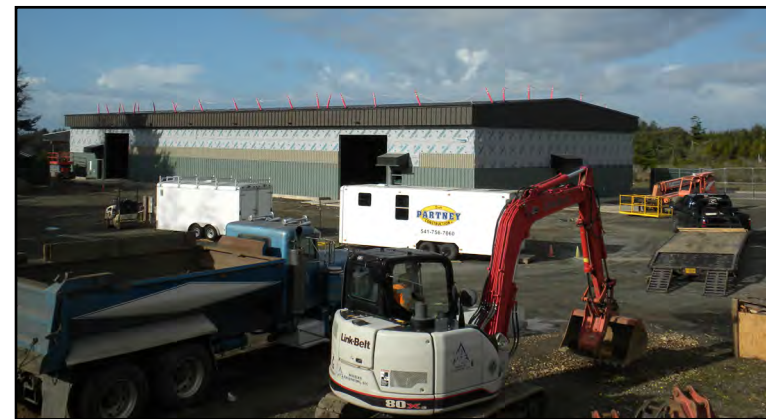
Early October: Siding begins to provide a finished look.
