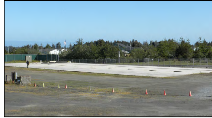
May: First step: A concrete slab.
