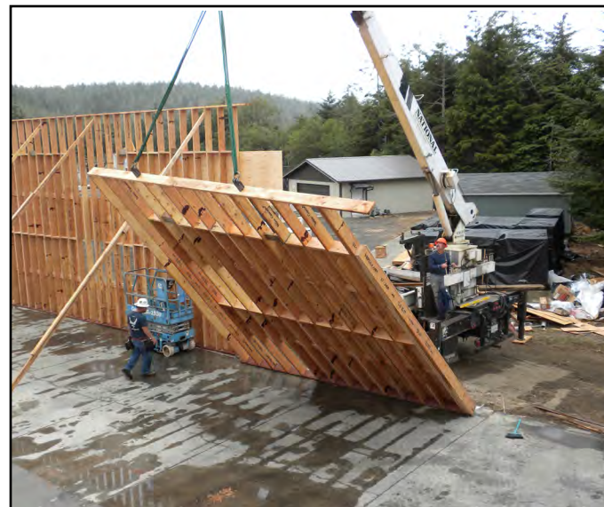
July: A crane hoists exterior framing into place.
