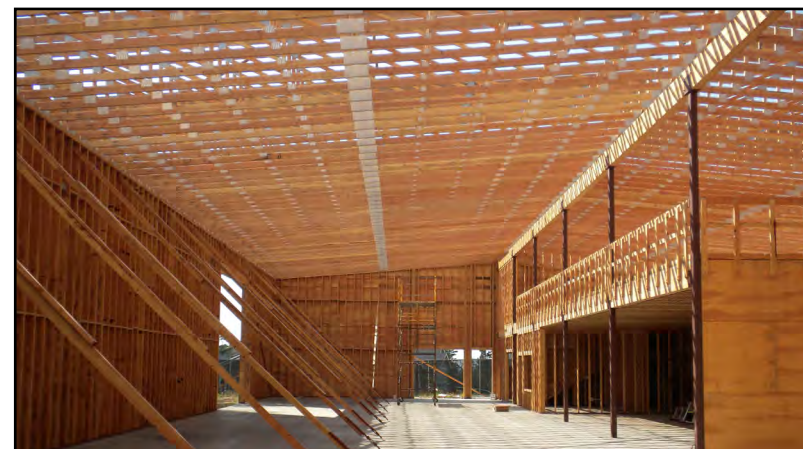
August: Roof trusses play a supporting role.
