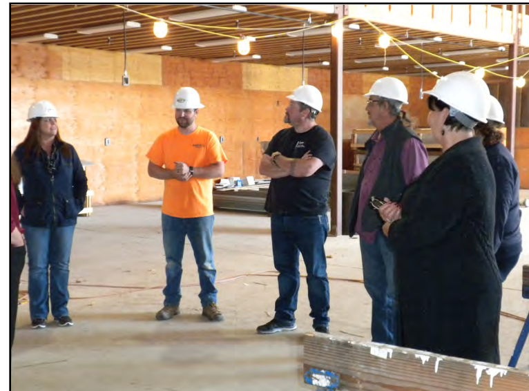
Oct. 16: Tribal Council tours the nearly complete building.
