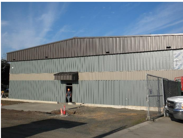
Nearing completion of siding installation.
