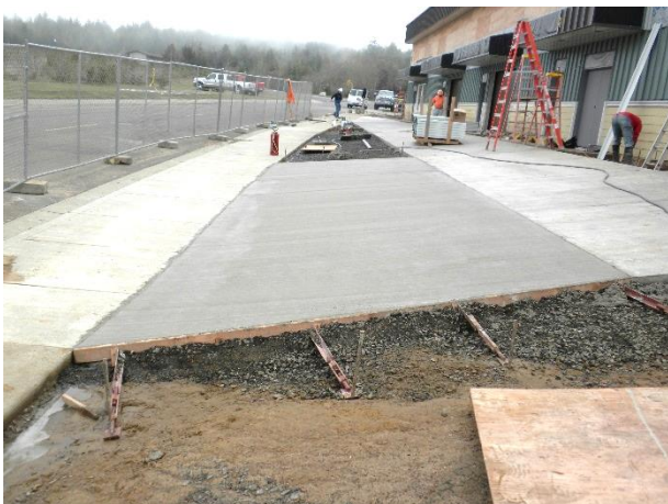
Pouring parking apron for rental units.
