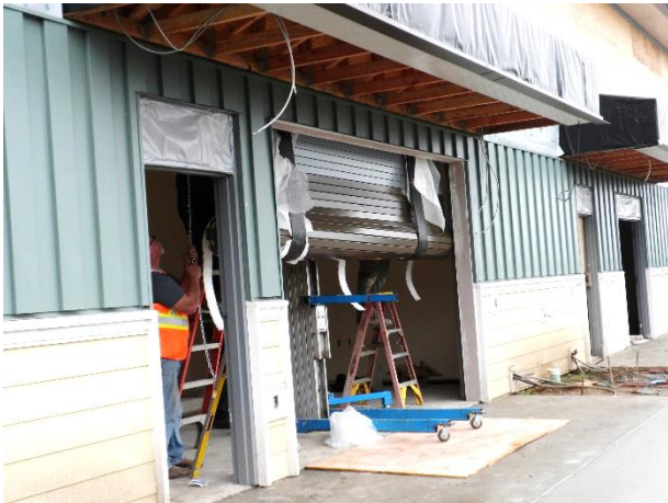
Installing roll up doors on rental units.
