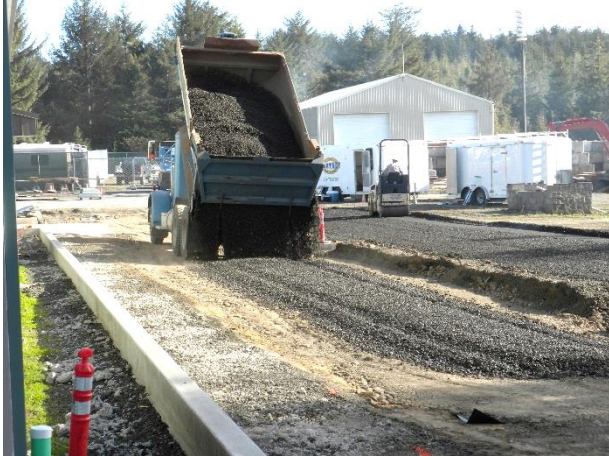
Spreading gravel on south side.
