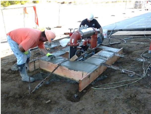
Pouring pad around fire system check valve.
