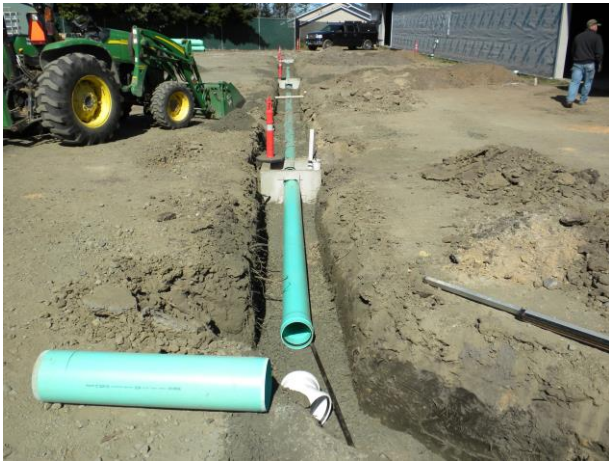
Installing site drainage system.
