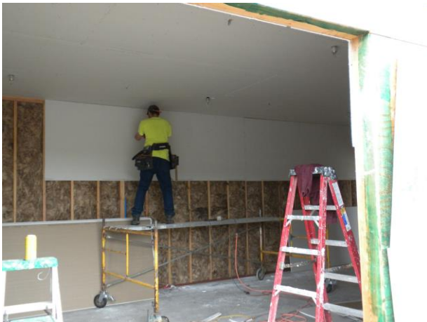
Hanging sheetrock in rentals.
