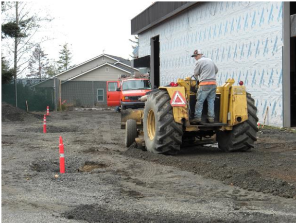
Site grading in progress.
