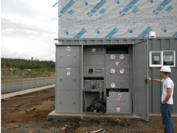
Meter base cabinet installed.
