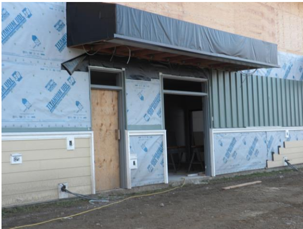
Installation of door canopies.
