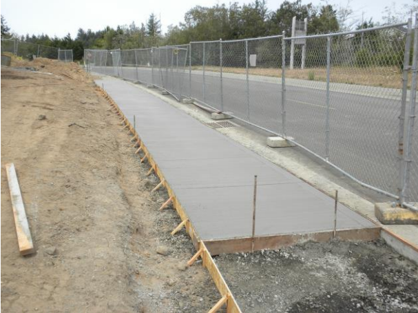
New sidewalk along Miluk Drive.
