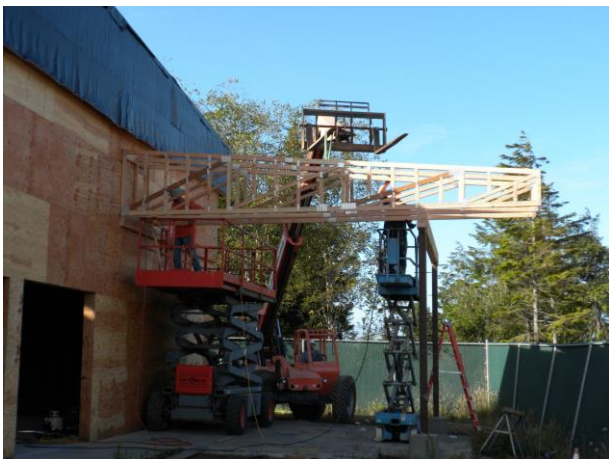
Washdown pad canopy.
