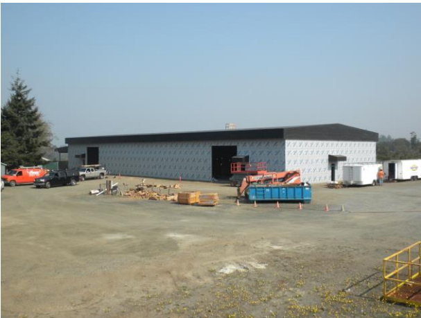
Weather resistant barrier installed.
