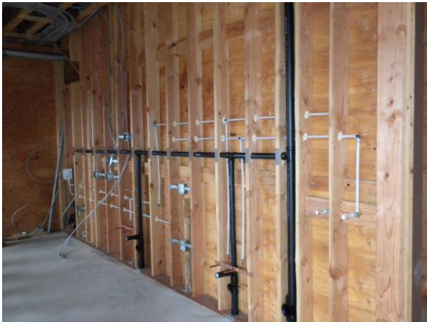
Plumbing and electrical rough in.
