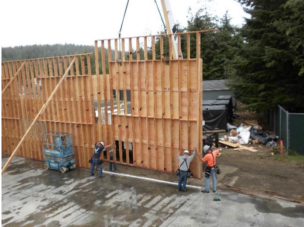
Raising the south exterior wall.
