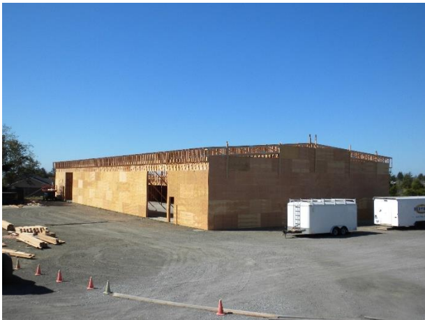
Exterior walls and roof trusses in place.
