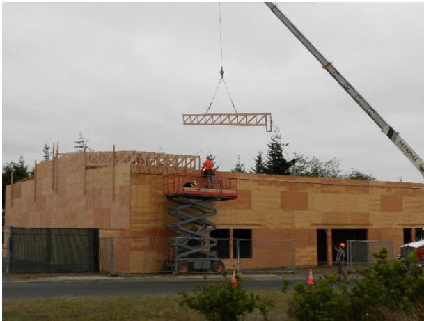
Setting the roof trusses.
