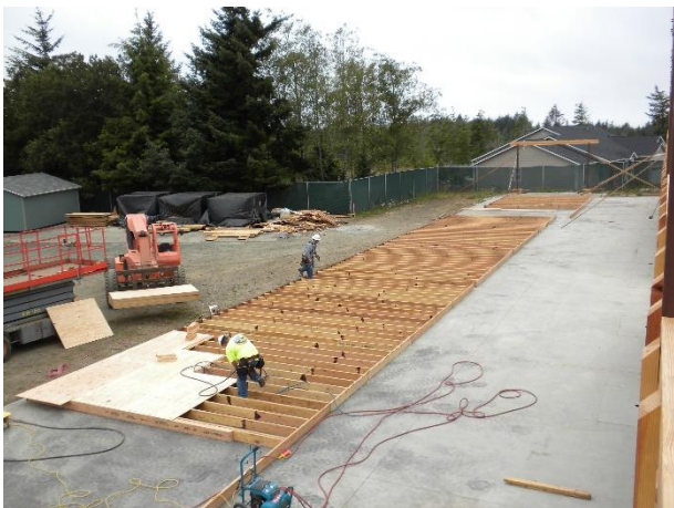
Framing the south exterior wall.
