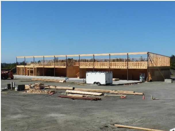
Roof beam installed.
