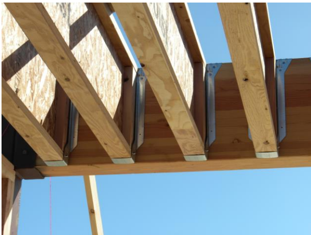
Mezzanine floor joists
