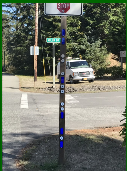
Reflectors have been placed on the sign posts at the bottom of Miluk Drive to assist traffic in locating the entrance to Tribal Lands easily at night.
